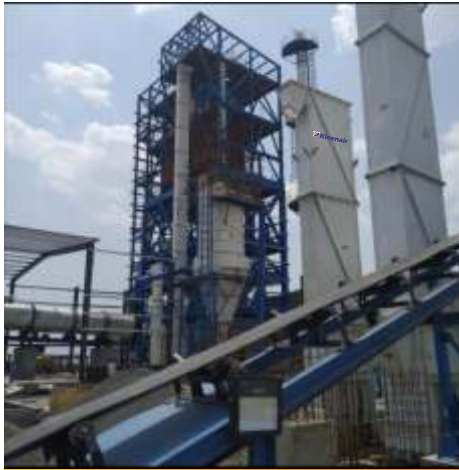
Plant under Installation
